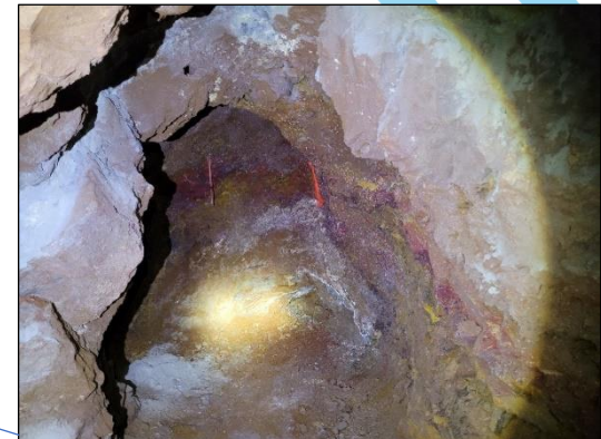
Orleans Mine - Eastern end of the 300' level
